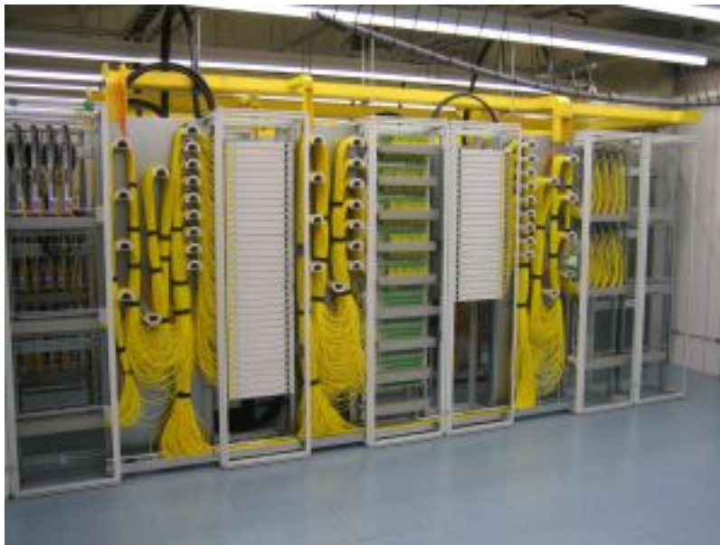
Fibre links at the point of presence (this one actually in Eindhoven)
